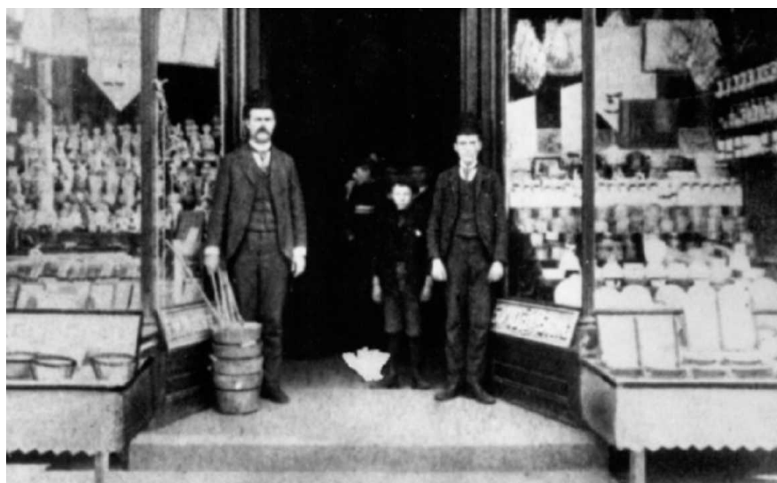
Fig. 1. Early Photo of the 19th-Century Storefront of F.W.
